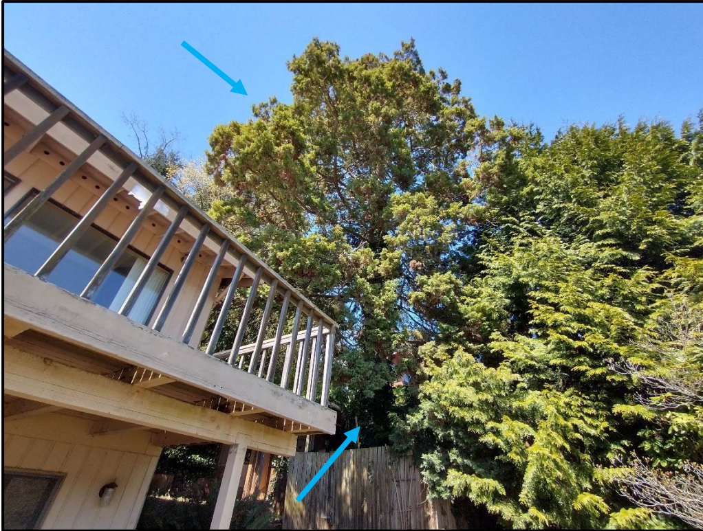
Photo 3. Tree 362, a Sawara cypress, directly adjacent to the shed proposed for removal. Demolition and construction activities adjacent to this tree should be monitored by an ISA certified arborist. Some clearance pruning may be required to accommodate site work.
